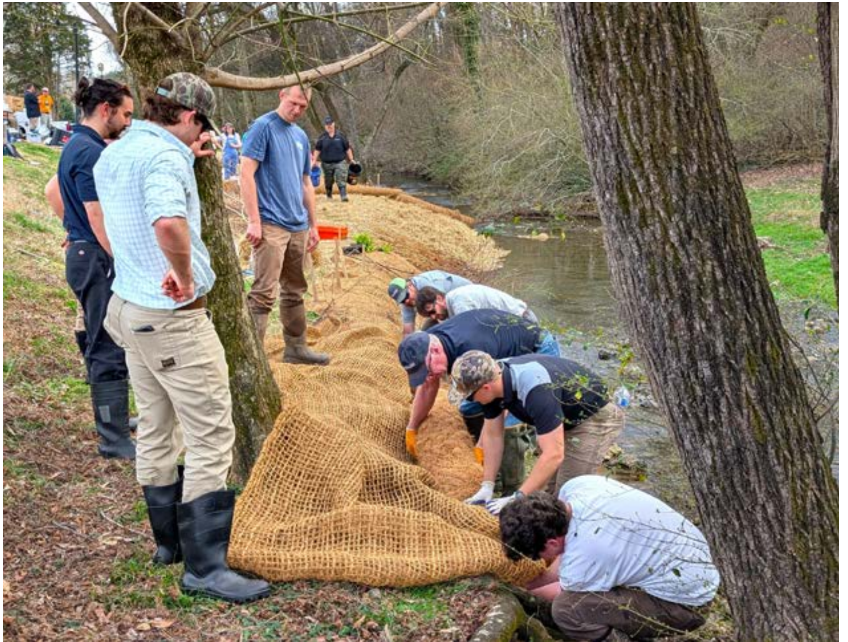
Local residents, professors and students from the University of Tennessee, and stormwater officials from Farragut, Knoxville, and Knox County spent an afternoon at Farragut’s Founders Park repairing riparian erosion on Turkey Creek. The workshop involved an educational session with presentations on how the mitigation project would work and then a hands-on component where participants got a chance to put what they had learned into action. (Photo by Farragut)
