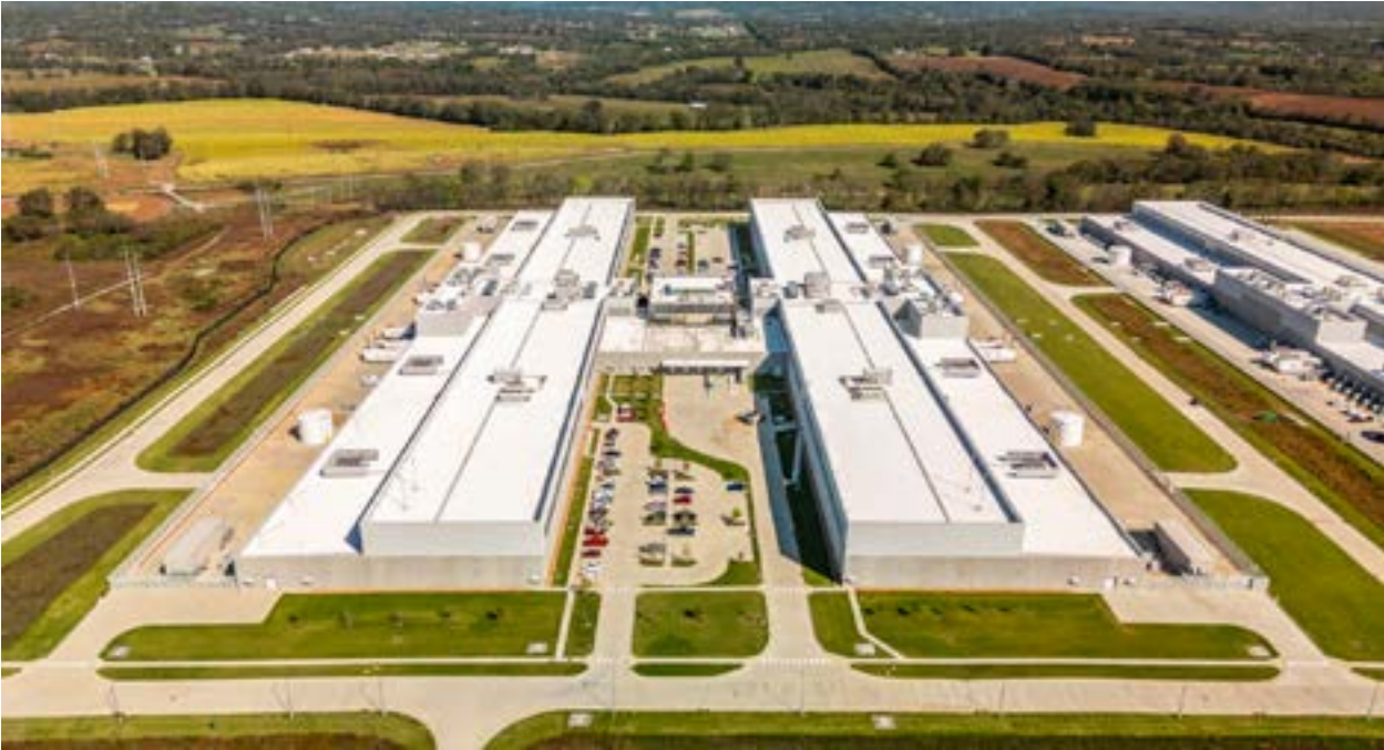
The same low tax rates, energy prices, and land costs that have driven other businesses to Tennessee have also cultivated the environment that attracts data centers, like the Meta Data Center in Gallatin pictured here, to the state. (Photo by Meta)
