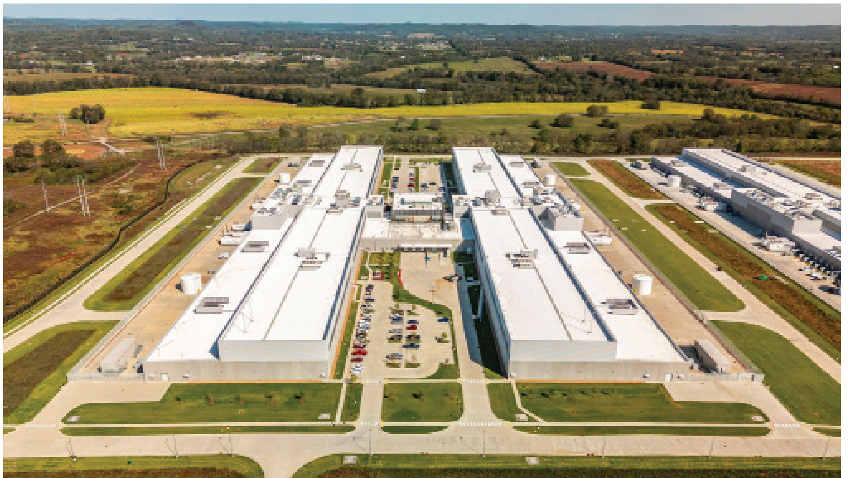
The new Meta Data Center in Gallatin is not only a major investment in the community but also represents more than $1.5 billion in investment in Tennessee.
