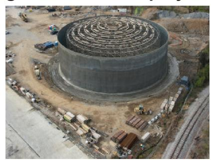
Gallatin Public Utilities is working to complete a project that will prevent strong rain events from overwhelming the sewer system and causing discharges of untreated water into Town Creek. The 10-million-gallon tank and pump "equalization basin" off Maple Drive will stagger the flow of water to the treatment plant and resolve the issue. The project was funded at \$12,200,000 and is expected to be complete in the summer of 2022.
