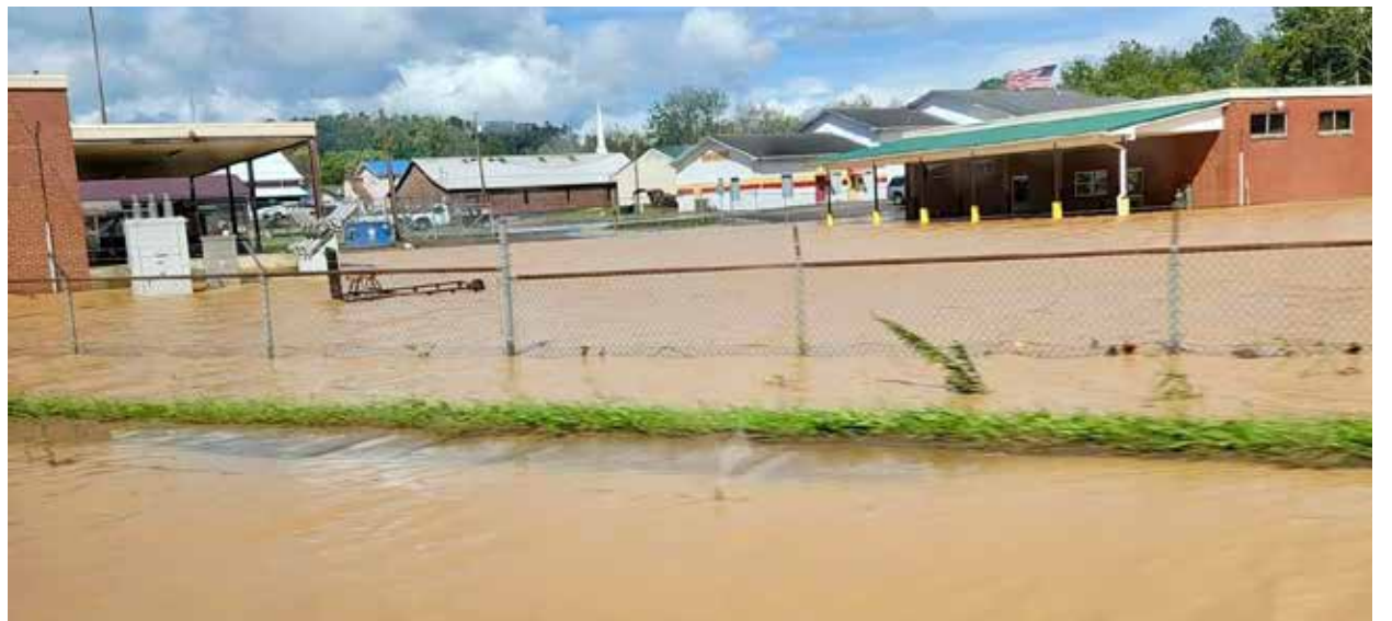
Floodwaters crest in downtown Mountain City near the local utility departments headquarters
