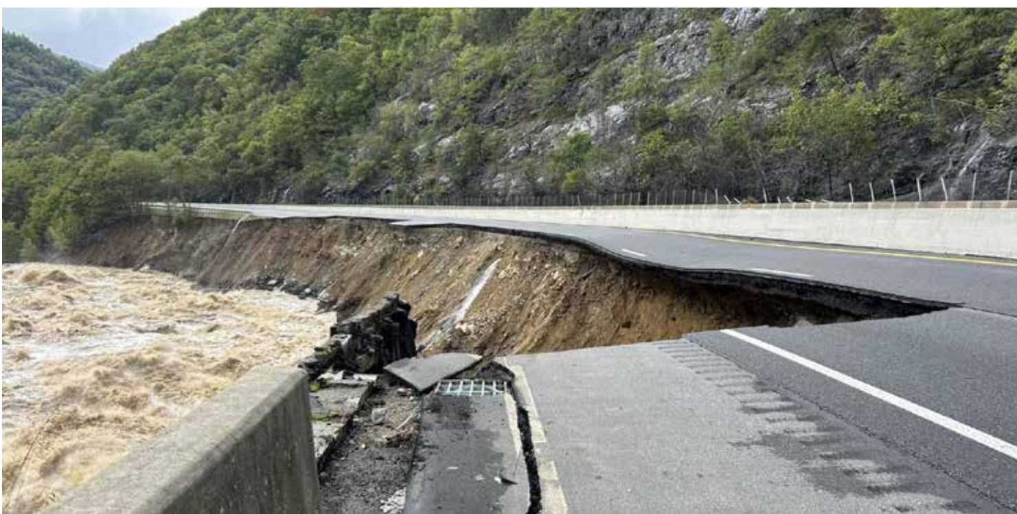
A portion of Interstate 40 is washed away about 3.5 miles from the North Carolina border. The interstate is closed from the Great Smoky Mountains National Park well into the state of North Carolina as a result of flood damage.
