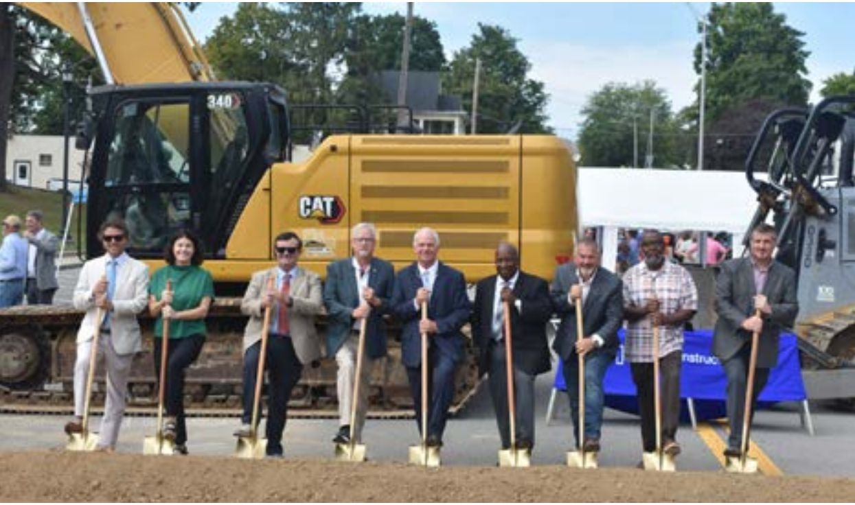
Officials with the city of Dickson have broken ground on a new 44,204-square-foot city center that will replace their existing 71-year-old municipal building. The new facility will consolidate the city’s police department, courtroom, and city administrative offices into a single facility. The project will also enhance public infrastructure in downtown Dickson, including road and surrounding sidewalk improvements. Construction is expected to be complete in March 2028. (Photo by Connor Butts/Dickson Post)
