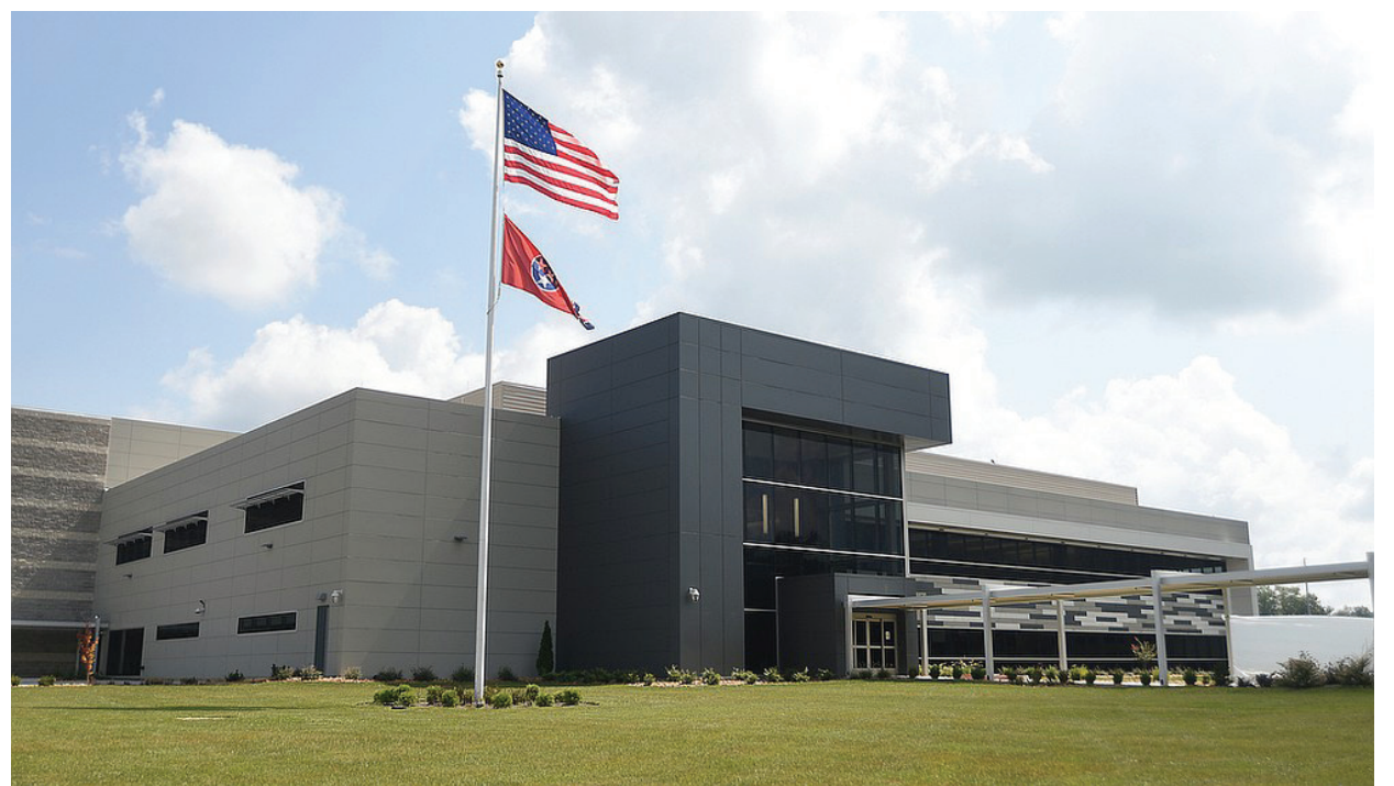
To meet with new demand, TVA recently opened this systems operation center just outside Cleveland. The new SOC will employ smart technologies to manage power grid operations more reliably and efficiently.
