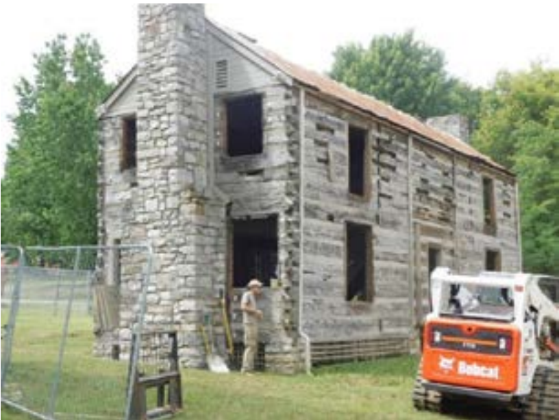
The original 200-year-old log cabin was beyond saving, but boards from it were reused to build the new pavilion.
