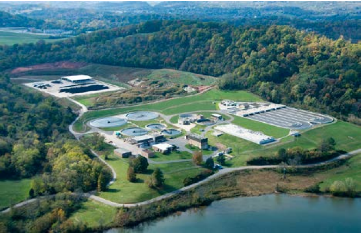
Electricity is not the only utility that is feeling the crunch from the state's growth in population and industry. As the state's water infrastructure ages, some water utilities have consolidated to maintain service due to decreasing populations. Other utilities are struggling to both maintain existing infrastructure while providing the new infrastructure population and business growth demands. hot data centers in particular use local water resources has become a hot button issue for many communities. (Photo by Maryville)
