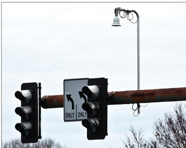
The city of Sevierville is upgrading its traffic technology, using equipment like this GridSmart fish-eye camera. The camera not only monitors traffic; it can count cars and keep track of what directions they are traveling in to help the city with data collection.
